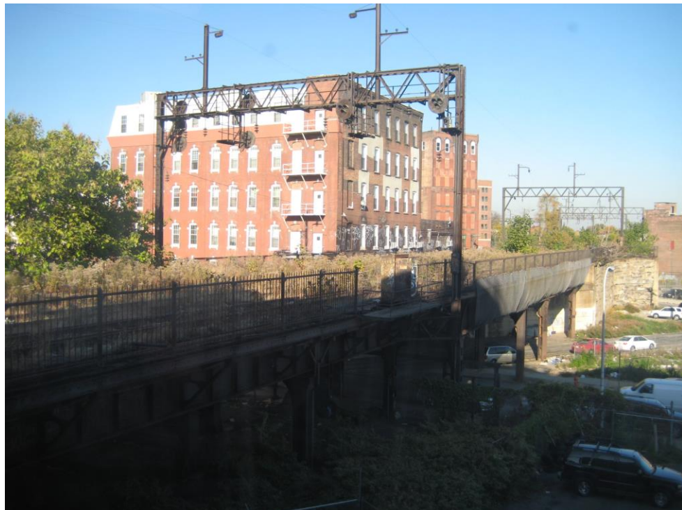
The Reading Viaduct
