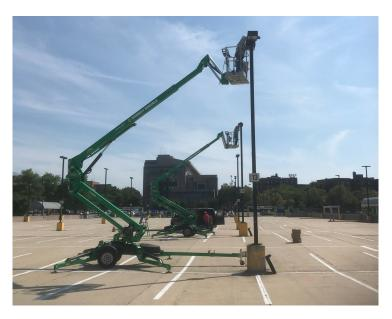
house electricians replaced all Parking Lot 14 light posts with a new LED," says Zeco Krcic (Facilities, Planning/Operations). "We went from 250-watt metal halide fixtures down to 78-watt LEDs."
