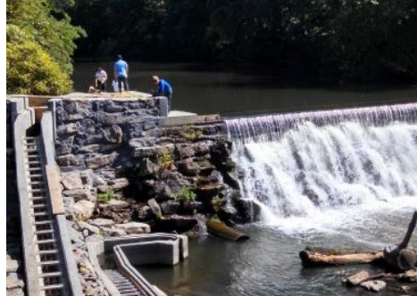
First fish ladder in the Bronx River. To date the ladder has passed modest numbers of river herring to go upstream to spawn.
